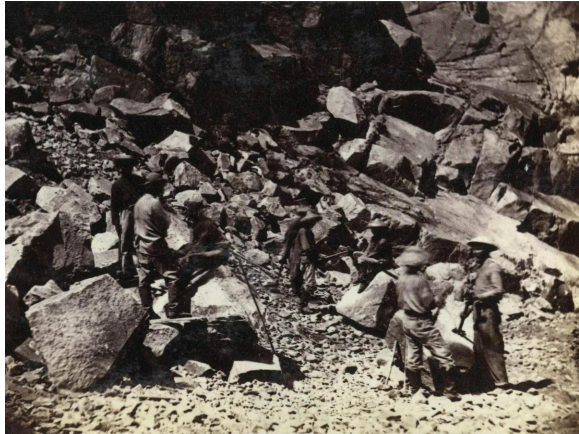
Chinese laborers constructing the Transcontinental Railroad circa the 1860s. Photo courtesy of Department of Special Collections, Stanford University Libraries.
